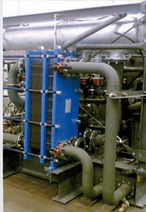
Cooling of hydraulic oil for high pressure air compressors in oil exploration.
